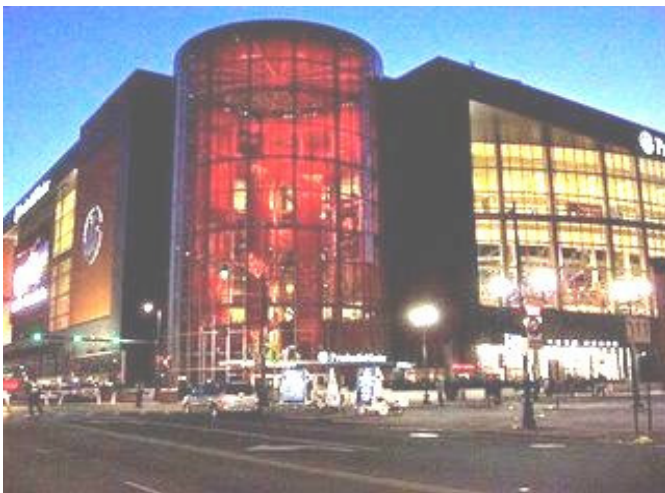
The “ROCK”, Prudential Center in Newark, NJ
